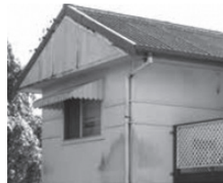
Asbestos Wall Sheeting
