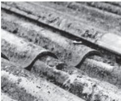
Super Six Asbestos Roof
